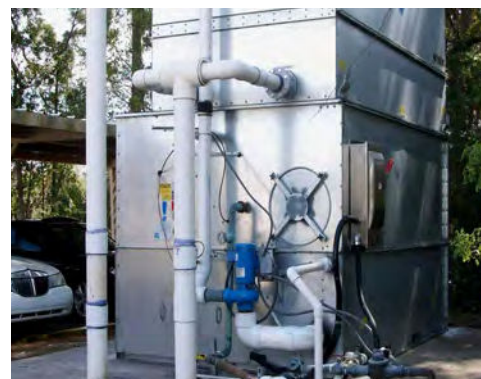
Standard Spray Water Pump
