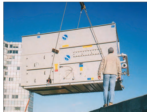
Single Piece Lift of a VFL
