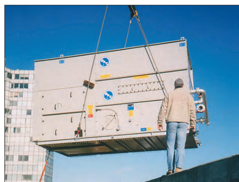
Single Piece Lift of a VFL
