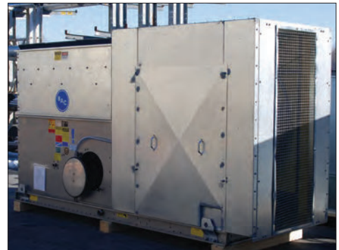
Intake Sound Attenuation
