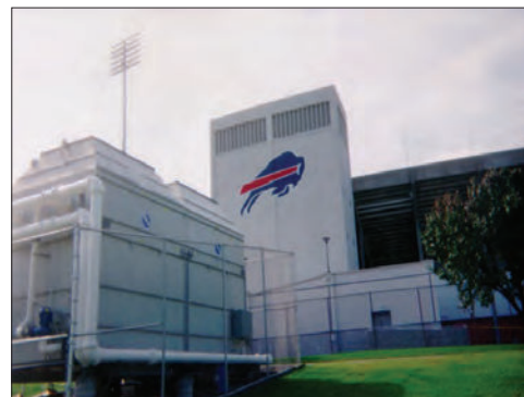
VF1 Closed Circuit Cooling Tower with Discharge Hood
