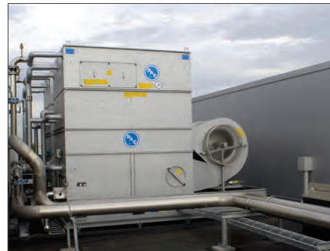
Standard Construction Installation
