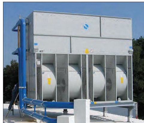
Thermosetting Hybrid Polymer Installation
