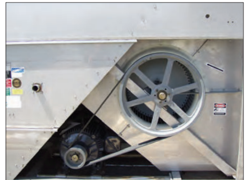
BALTIDRIVE® Power Train Fan System
